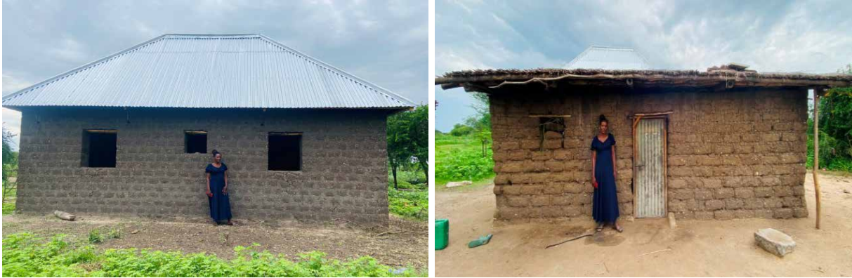
Income attainment enhances Gaudensia Mange's achieved to improve the house; from grass thatched (left) to iron roofed house(right); (Photo taken by; Raiya Masoud –TCRS staff);
