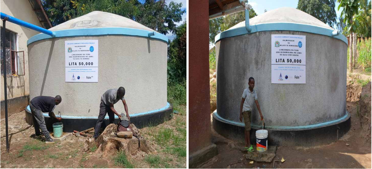
RWH tanks at Kiroka Dispensary and Vuleni Primary School.
