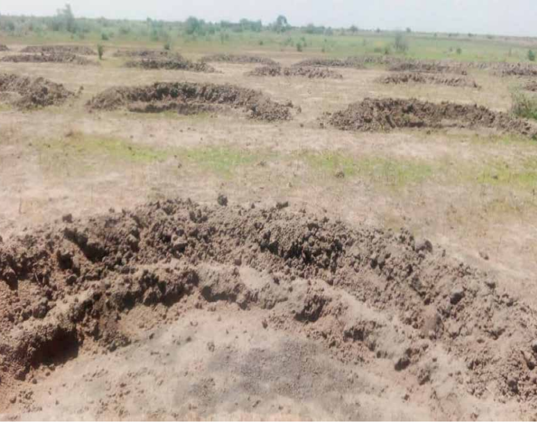
Regreening or vegetation restoration by rainwater harvesting half-moon bunds method at Ngeme village- the left photo in October and right photo in December 2024; (Photo by Emmanuel Sanyenge-TCRS staff)
