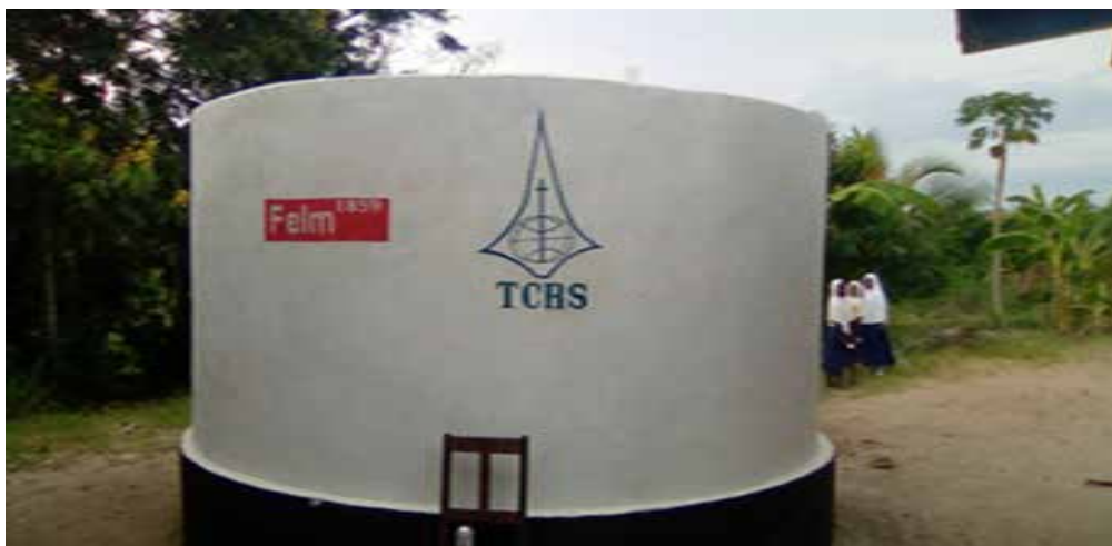
Water tank supported by TCRS at Chapita primary school
