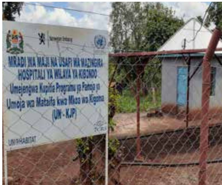
Pump house in a borehole drilled to increase supply of water at KDH
