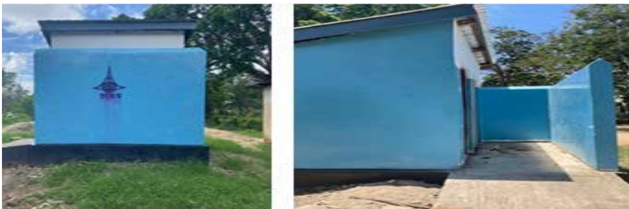
Ventilated pit latrine at Somanga Simu primary school
