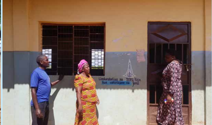
Classroom rehabilitated by project at Juhudi Primary school
