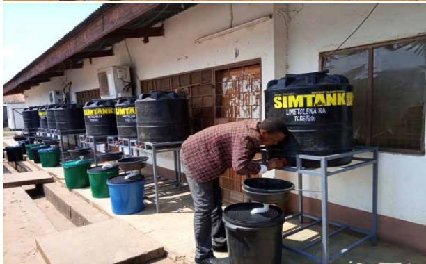
Hand washing machines with sim tank supported for WASH at police station mikese and for business centers at Morogoro municipal
