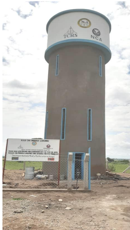
Photo: 45 M 3 Raiser storage tank after construction completion.
