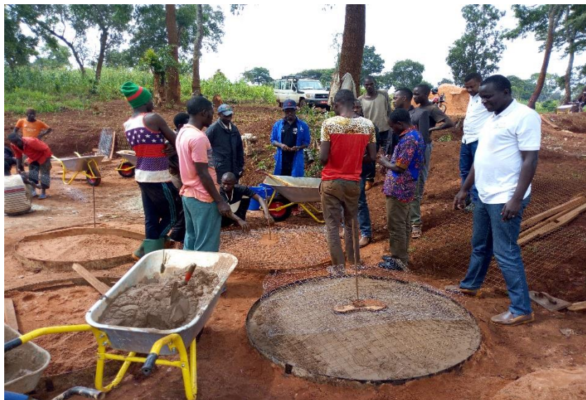
Photo: Production of doomed mold for latrines
