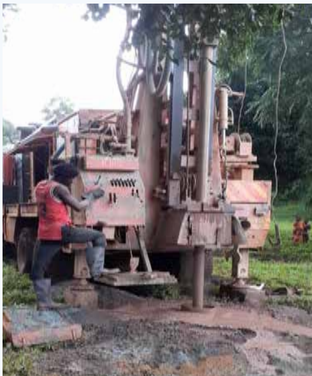
Drilling of a borehole to serve Kibondo District Hospital
