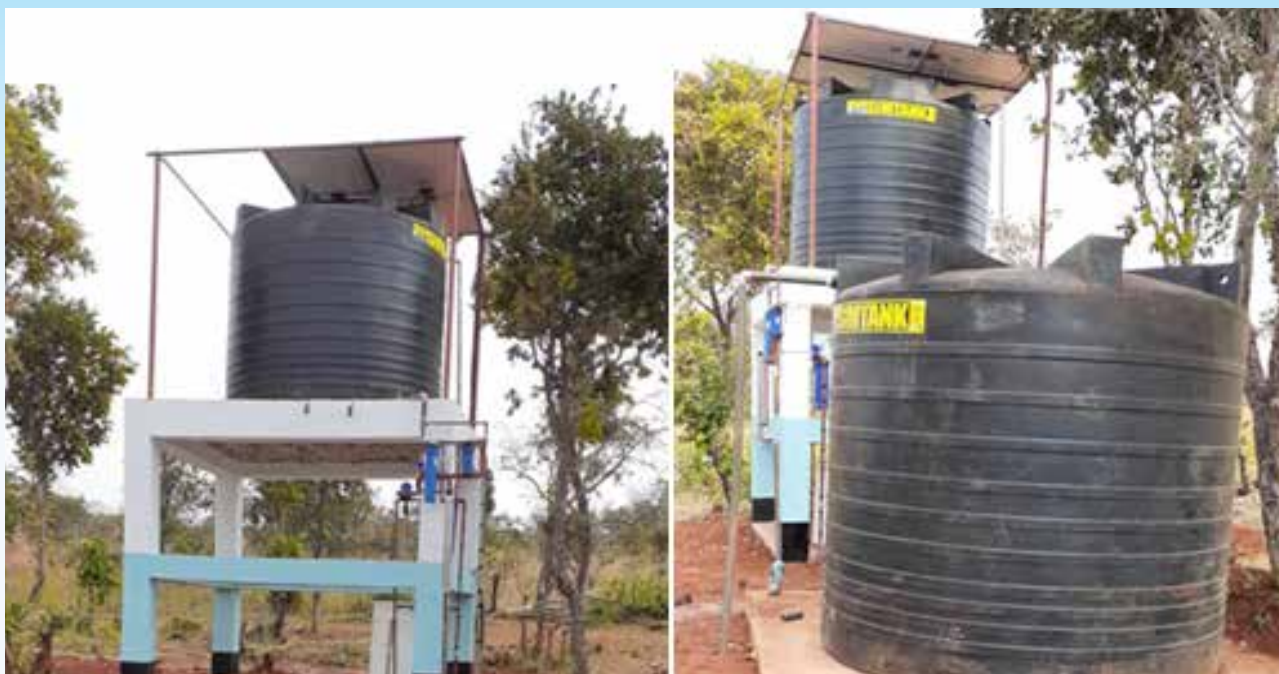
Complete installed water storage unit and pumping system at Gwanump Health Center
