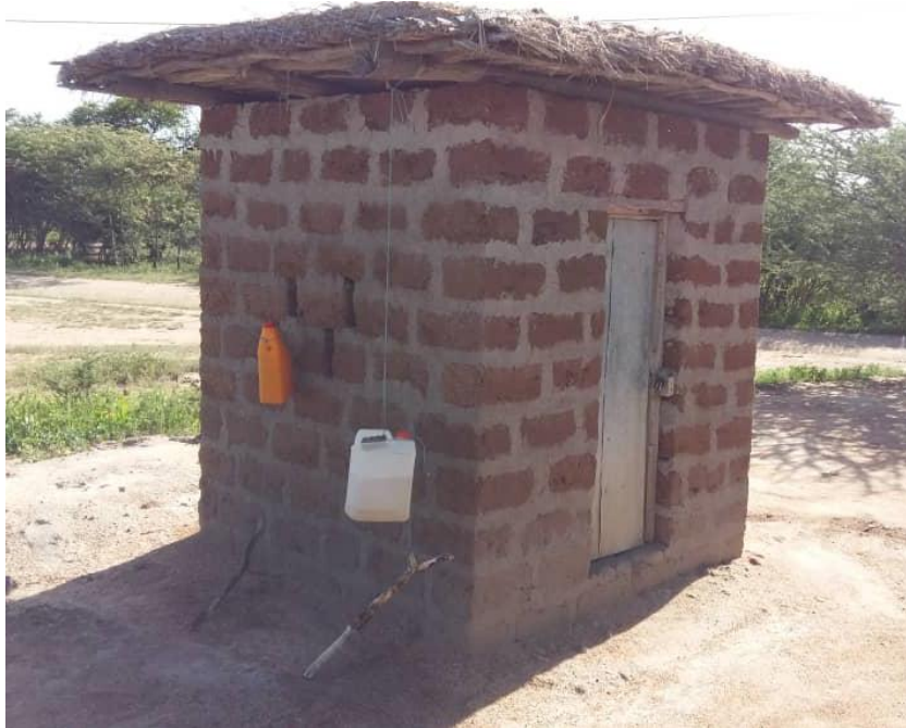
Photo: Sanitation and hygiene enhanced by household pit latrine with hand washing facility-tippy tape technology
